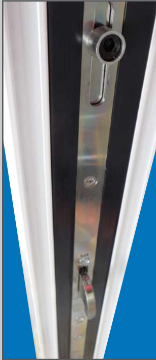
View of lower hook bolt and cam
